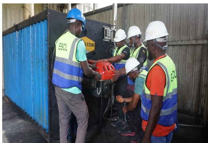
Maintenance (Boiler) Unit
